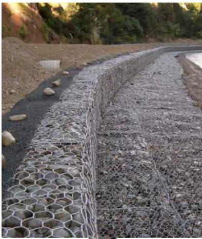
Protect the river bank
