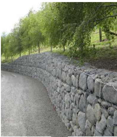
Protect the roadway
