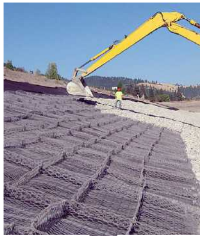
Soil erosion control
