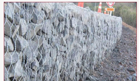
Stronger coastal slopes with gabion meshes
