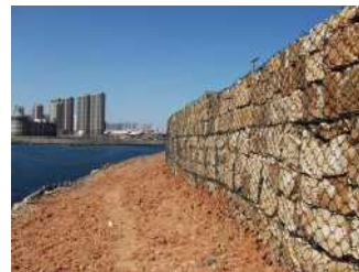
River Bank Protection
