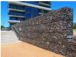
Office Building Feature Wall
